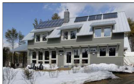
Gordon Chibroski/Staff Photographer The green show house on Cranberry Ridge Road in Freeport has solar panels and collectors, a metal roof and large, energy-efficient windows.
